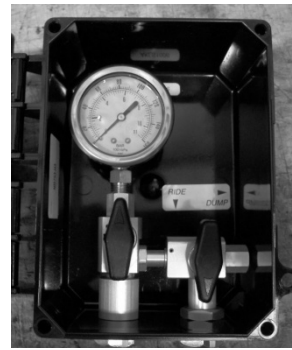
Figure 55 - Dump valve used with air gauge
